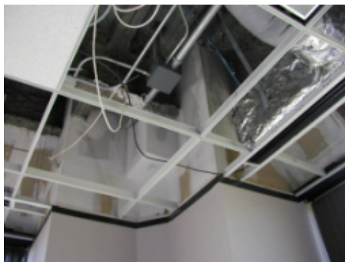
Photograph 3: Retrofit of Closure
