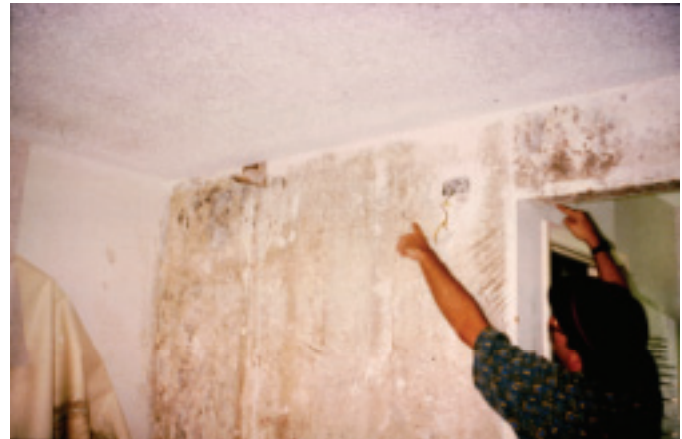
Photograph 5: Hotel Room Flow Path Part II
